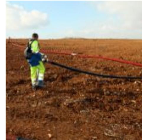
Hersin-Coupigny, SITA North (France) - ISDND, provisional biogas monitoring network before final acceptance
